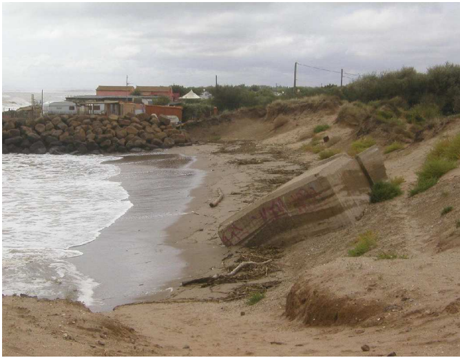
Erosion vs protection © CAHM
